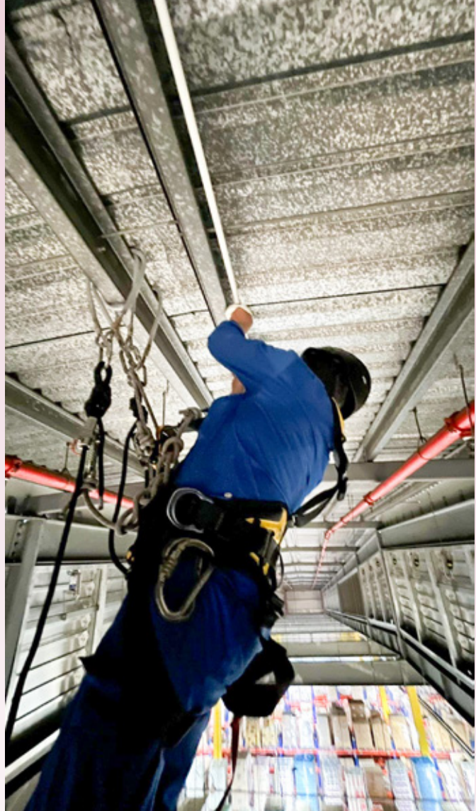
Our own UEMS Height Specialist, Majin Bin Kansirung installing Smoke Detectors via Rope Access Rappelling
